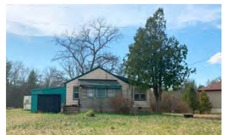
(Above) Photograph of the Sarge Johnson Homestead & Paddock today as observed during the field survey.
