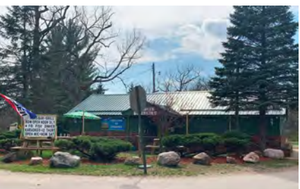
(Above) Photograph of the Red Rooster today as observed during the field survey.
