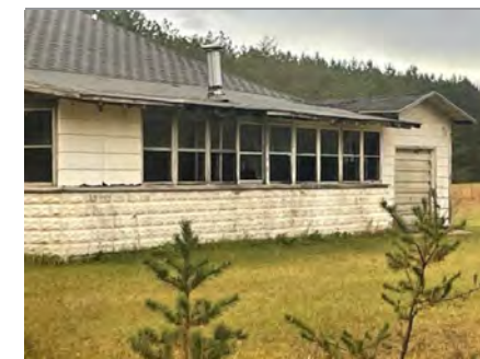
(Above) Photograph of the Club El Morocco (Courtesy of Chris Kingdom-Grier)
